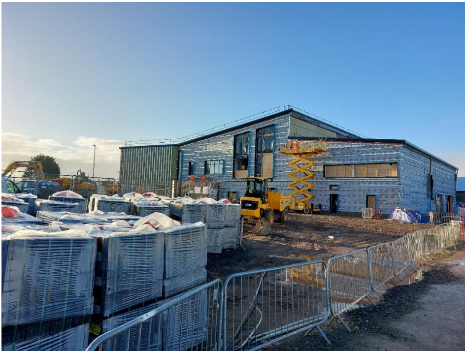
East elevation under construction
