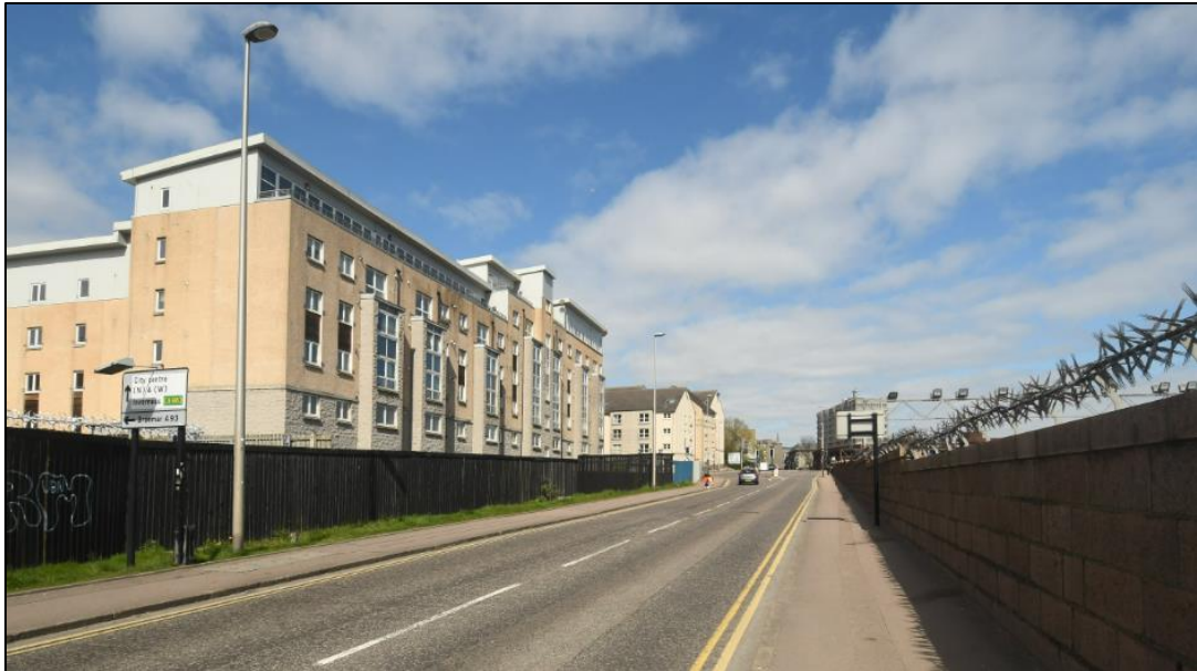
South College Street looking towards Wellington Place prior to works start
