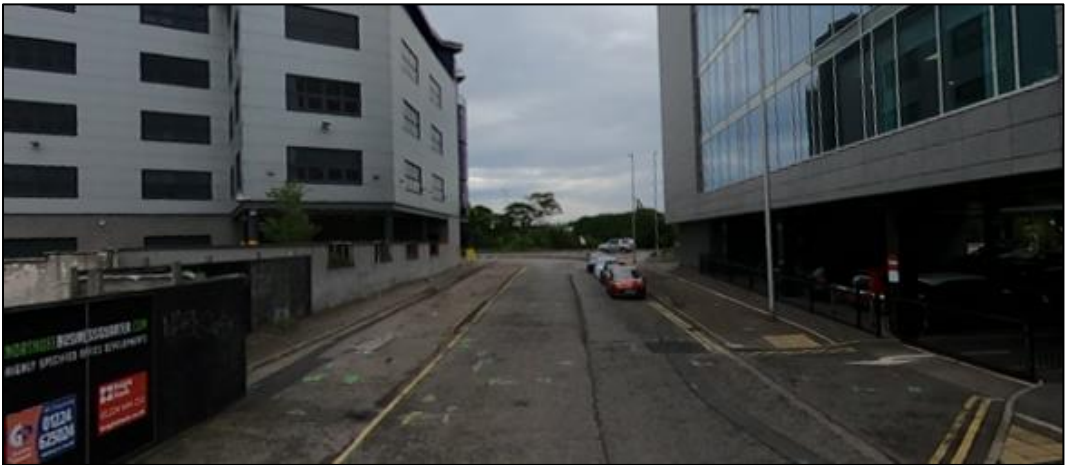
Palmerston Place looking toward North Esplanade West prior to works start
